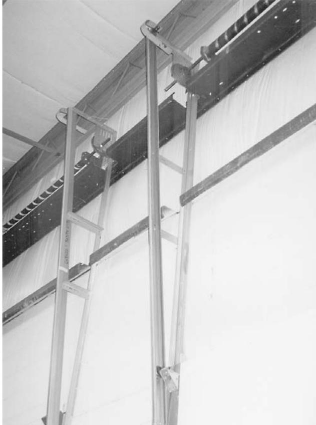
**FIGURE 10.9** These overhead door jambs are not supported at the top by anything other than the girts—which were cut to allow for the jamb installation.
